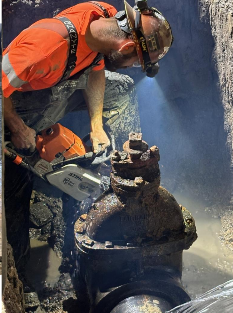
Cutting Out the Old Valve
